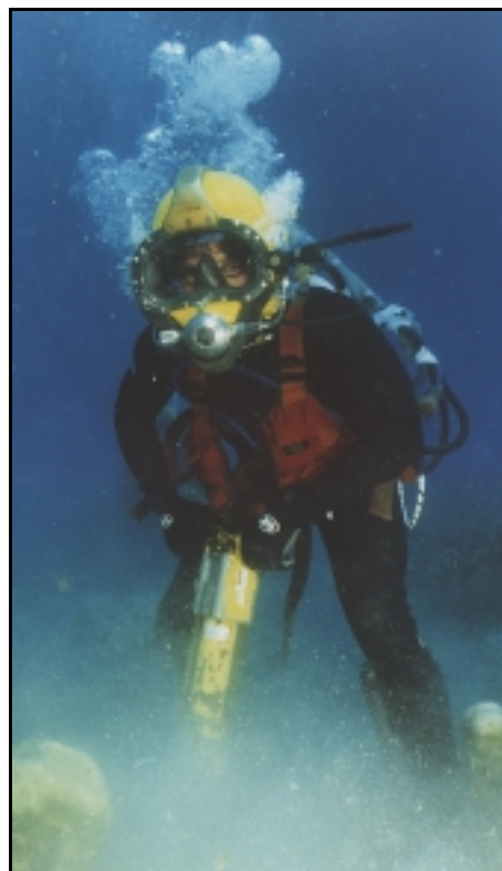
Figure 6-4. Underwater Construction Diving.
